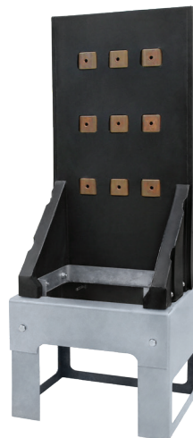
Blanking plugs cover unused live parts
